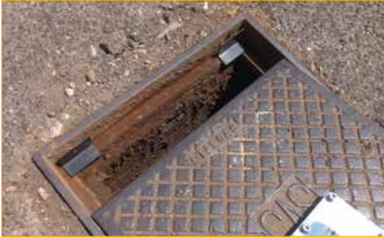
Shims positioning between cover and frame.
