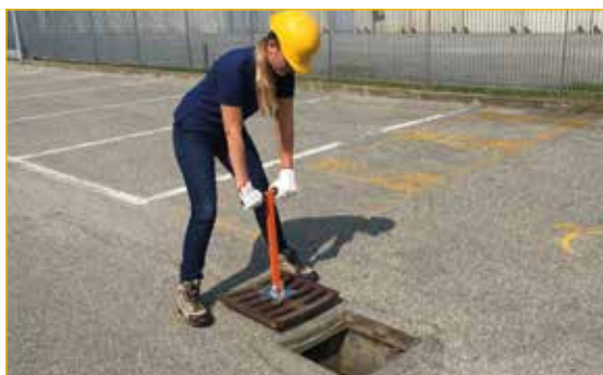
Opening manually light/middle weight lid.
